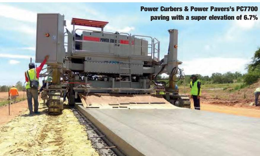
**Power Curbers & Power Pavers's PC7700 paving with a super elevation of 6.7%**
